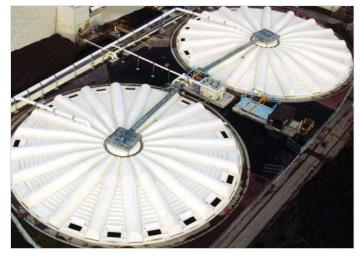
Gravity thickeners thicken primary sludge.
